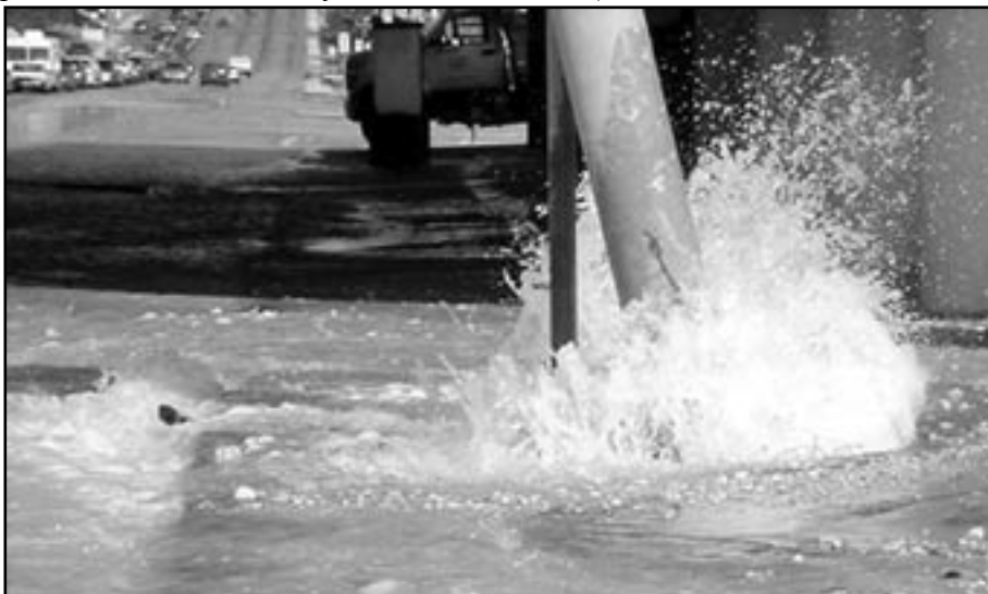
Most main breaks are not as spectacular as this one that occurred in June, 2004 at Bandera and Loop 410, snarling traffic for hours; water or wastewater system breaks are occurring all over town at record-high numbers because of the dry weather. Call 704-SAWS if you see one.
